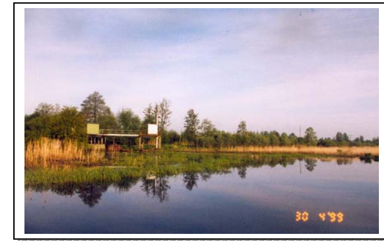
Station de pompage
